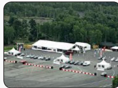
Helicopter view of C.E.R.A.M. test track
